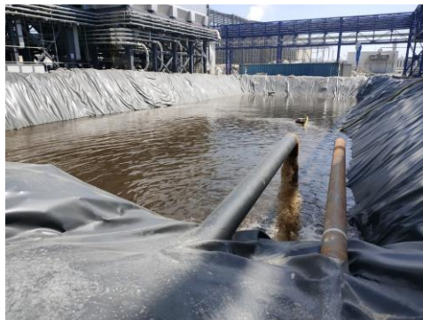
Figure 4 — Start of flushing: dirty water discharge to temporary settling pond (high suspended solids).
