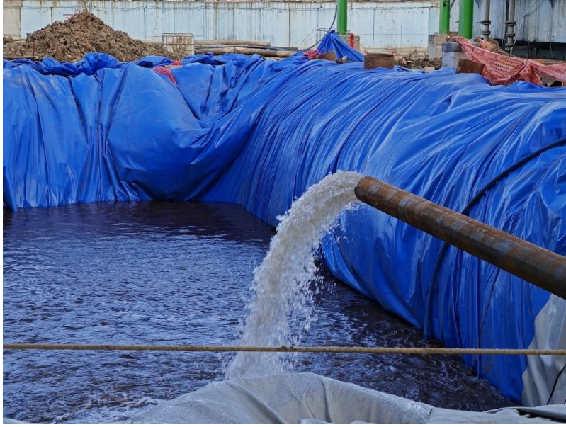
Figure 5 — Flushing completed: clear water discharge (separate project).
