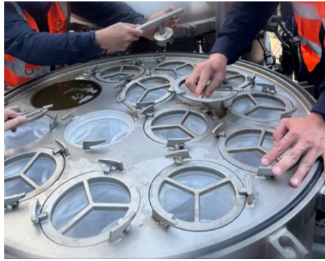
Figure 2 — Stainless steel multi-bag filter housing.
